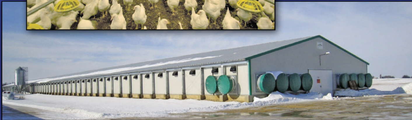
Complete tunnel ventilation control
