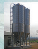
Feed silo weighing
